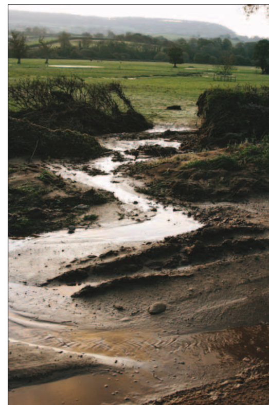
Figure 12. Looking southeast from the unclassified road just north of Fluxton. Note the section of hedge and supporting earth bank which has been removed by the floodwaters.
