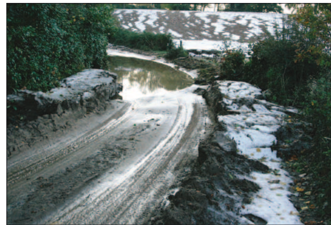
Figure 14. Looking south along the unclassified road to Fluxton, about 0.5 km south of Ottery St Mary, where a small stream crosses under the road. Note the removal of the hedges on the west side of the road close to the course of the stream.
