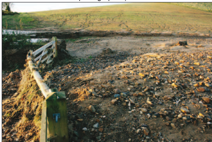
Figure 9. looking south over fields just north of Bishops Court. The debris on top of the gate show that the floodwaters must have been over 1.2 metres deep at their height. Note the large accumulations of hail on the upslope side of the hedges bordering the road, on the far left of the photo. The larger rocks exposed in the field were at least 30 cm long.
