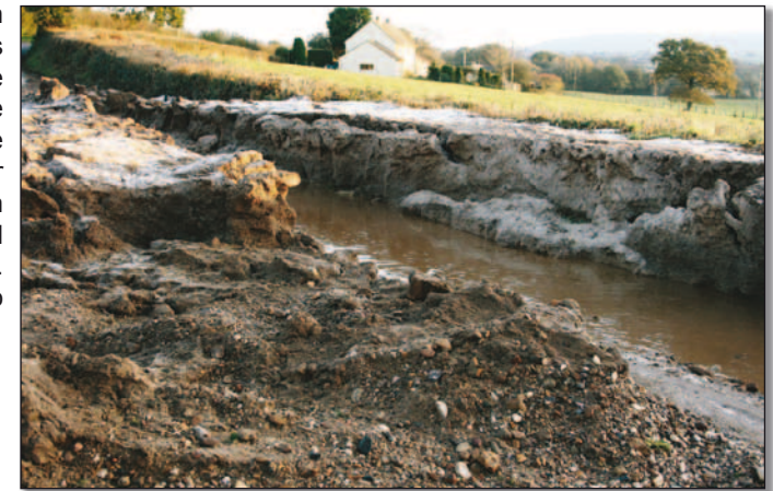
Figure 8. Looking northeast, across the unclassified north-south road just north of Bishop's Court.
